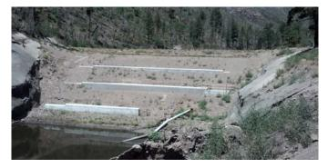
provide a load bearing footing at several elevations across the downstream face of an embankment dam. In this application we're constructing a roller compacted concrete spillway over the embankment, so it has some similarities to the Pueblo Levee. This spillway will pass the probable maximum flood so is more robust than is likely needed for the Pueblo Levee.
