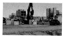
Thick to 20'x20' ID x 18" Thick. The vaults were installed up to 25' in depth. On Buckley AFB we installed 27 electric and communication vaults with bases ranging in size from 8'x12' ID x 10" Thick to 12'x14' ID x 12" Thick. The vaults were installed up to 15' in depth. All vault installation involved moving the vault bases, wall sections and lids around a congested construction site and setting them in excavations.
